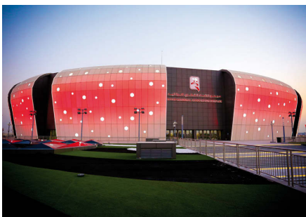
Qatar Handball Stadium illuminated with Square Grazer®
