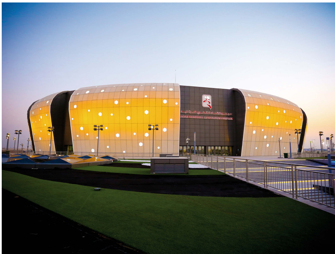
Qatar Handball Association Complex, Doha, Qatar
