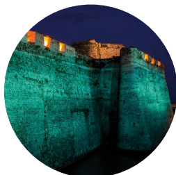
10 Royal Walls of Ceuta Ceuta, SPAIN
