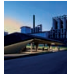
Zeche Zollverein Essen (Germany) Project: Lighting Design: Engineer Büro Paulus Essen, Herr Gräf Photography: Linea Light GmbH
