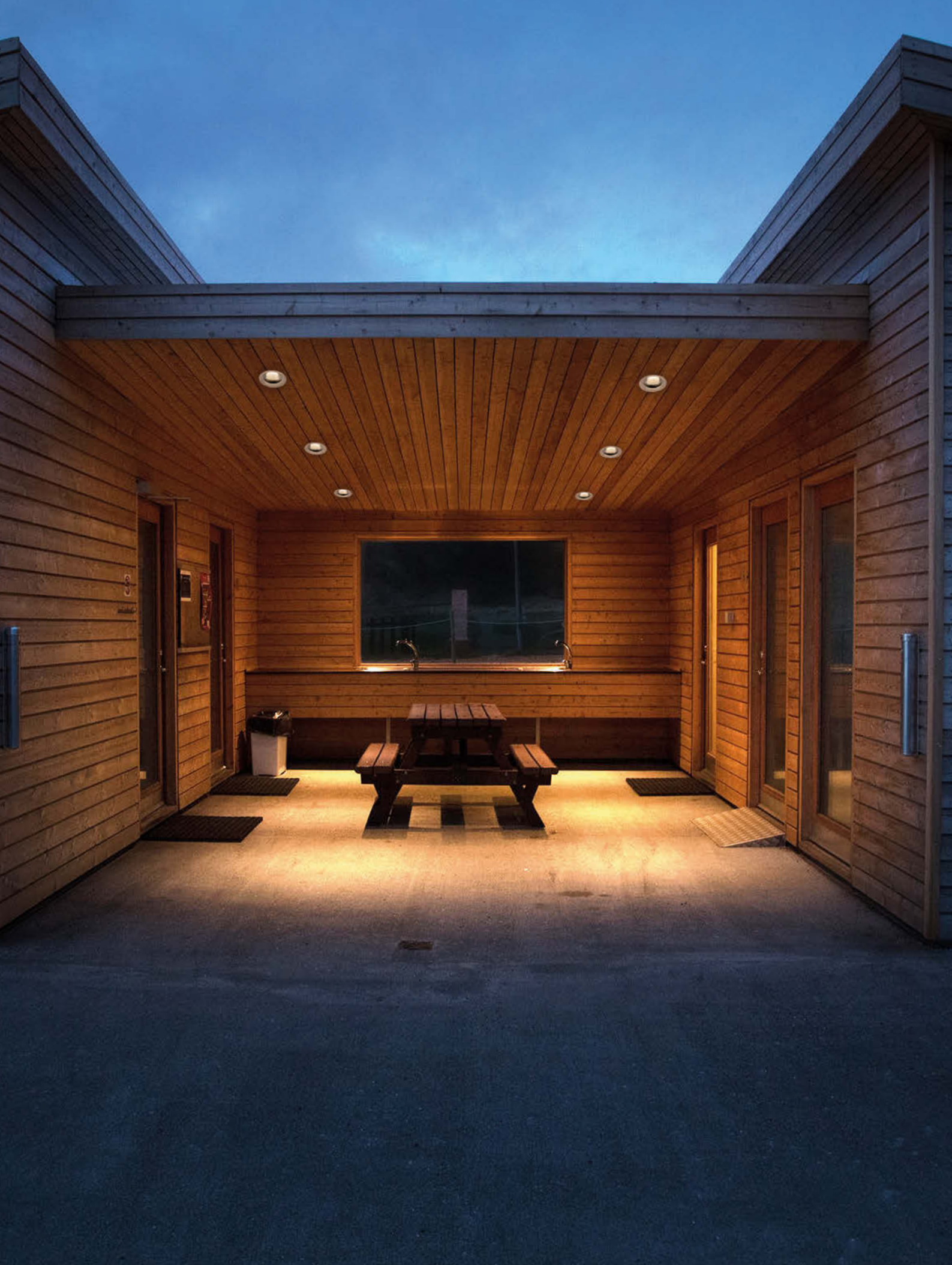
OUTDOOR - FIXED DOWNLIGHTS
