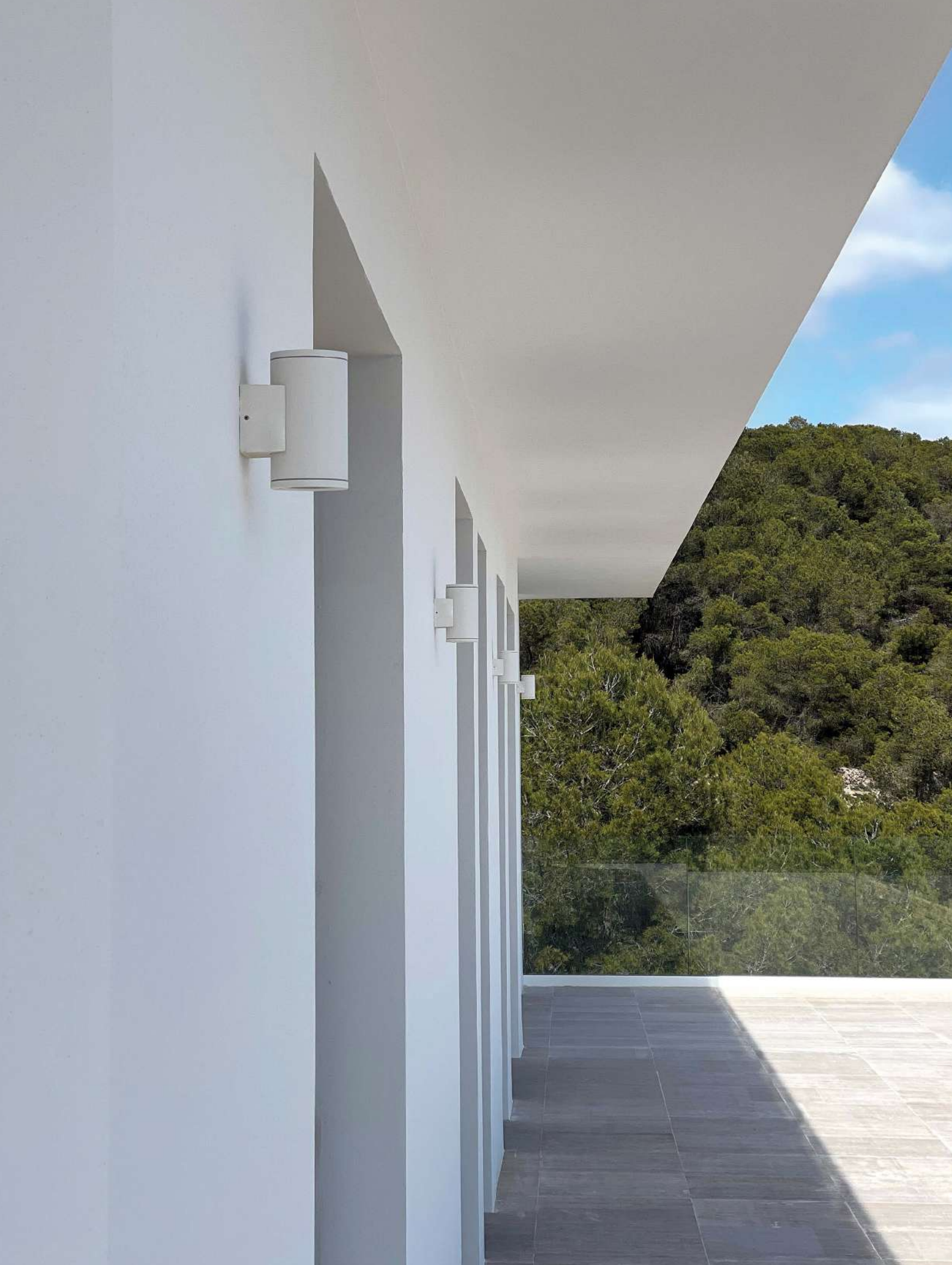
OUTDOOR - WALL FIXTURES
