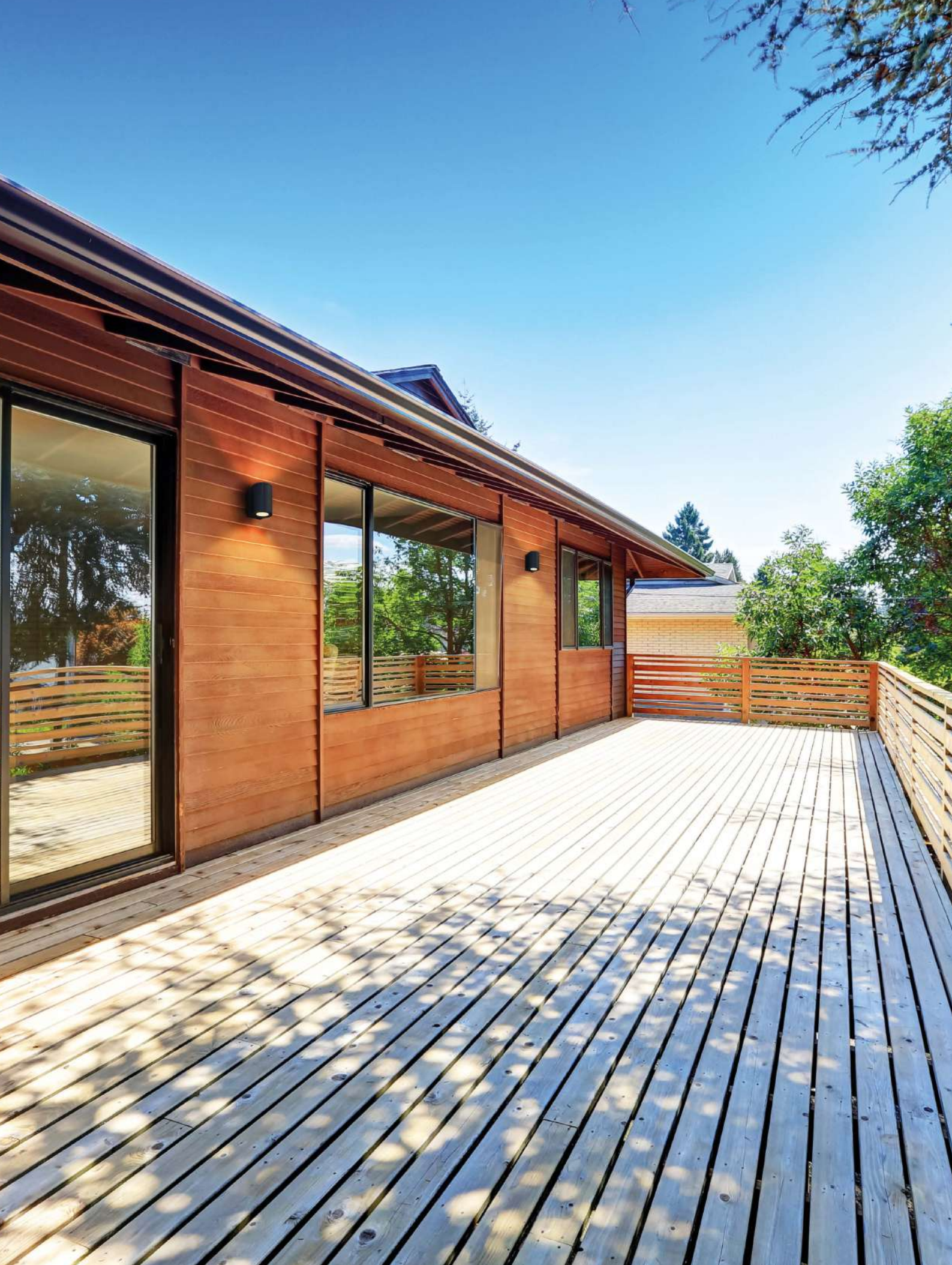
OUTDOOR - WALL FIXTURES
