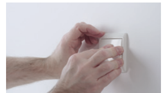
04 Mount the cover of the pushbutton.
