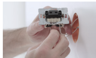
03 Connect the DALI PCU to the pushbutton.
